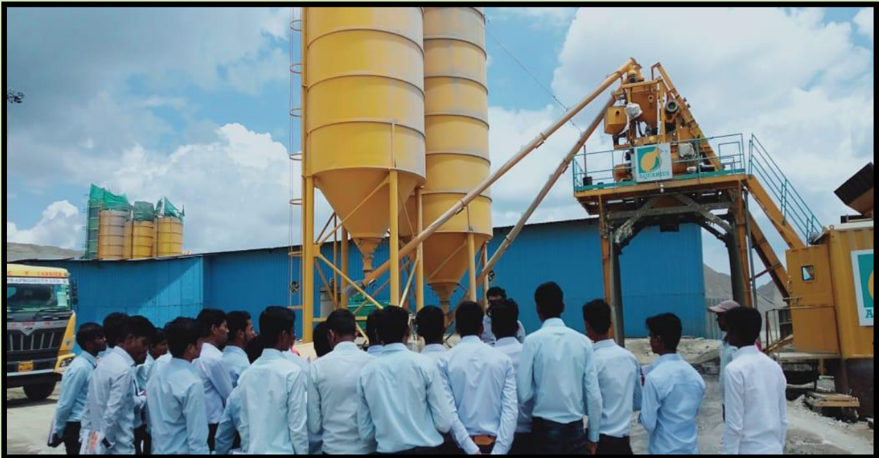
RMC Plant, GRIL InfraprojectsPvt ltd, Valsang, Akkalkot.
