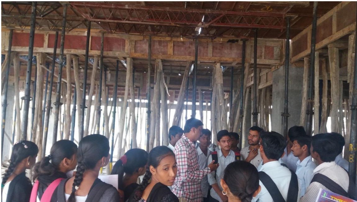
CONSTRUCTION OF MULTISTORIED BUILDING
